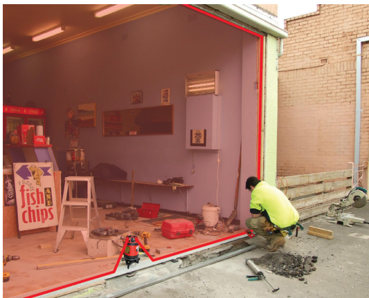
Laser receiver LRMULTI is used to pick up the lines as all line lasers are difficult to visually see when used outdoors. Picture shows a graphical representation of laser lines
