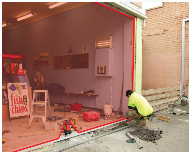
Laser receiver LLR705 is used to pick up the lines as all line lasers are difficult to visually see when used outdoors. Picture shows a graphical representation of laser lines
