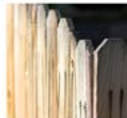
Fencing, Alignment & Height
